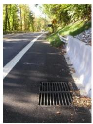
**BAD NEWS:** The new bridge on Maryland 450 (Defense Highway) over the headwaters of the South River has two of the notorious 'bicycle trap' drainage grates installed on the westbound shoulder – one just at the beginning of the newly paved area, and one (shown) after you pass over the bridge.
